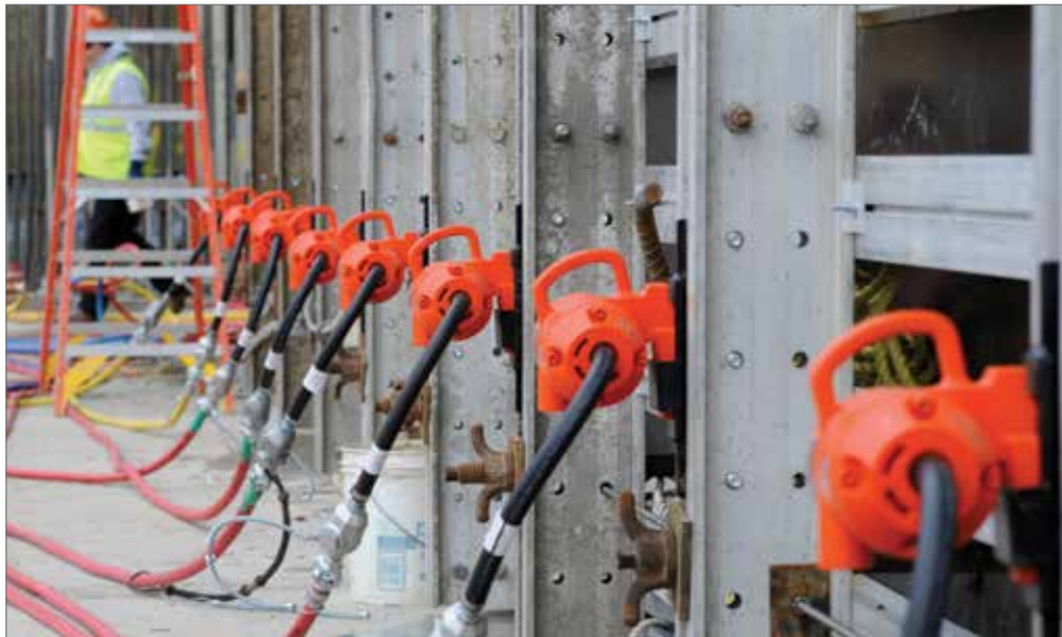
VIBCO Vibrators are right at home in concrete applications whether it be for columns, walls, slabs, foundations, or precast. Below, our Model SVRFS (page 30-31) with Stik-It™ Mount (page 65) is being used for bridge repair in RI, and at left, mounted onto a concrete column form. Above, our SVRWS (page 30-31) is being used with a UWF bracket for excellent transfer of vibration. VIBCO has brackets that will work well with any concrete form including wood.
