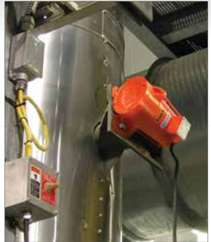
Above: The SFC Model shown on the hopper with a special heat mount (consult factory) is ideal for use in this high heat environment.
