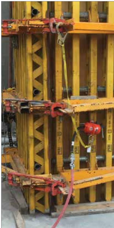
VIBCO Vibrators are right at home in concrete applications whether it be for columns, walls, slabs, foundations, or precast. Below, our Model SVRFS (page 30-31) with Stik-It™ Mount (page 65) is being used for bridge repair in RI, and at left, mounted onto a concrete column form. Above, our SVRWS (page 30-31) is being used with a UWF bracket for excellent transfer of vibration. VIBCO has brackets that will work well with any concrete form including wood.
