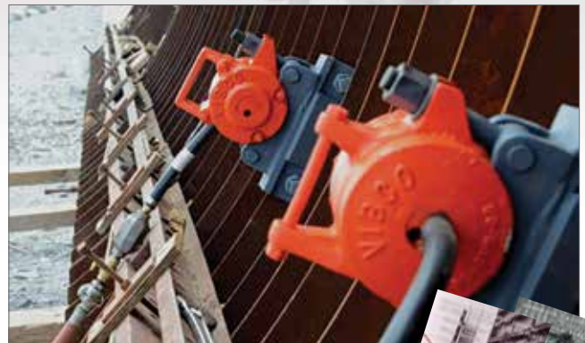
The SVRL Units shown here are being used to strengthen a concrete retaining wall. The Lug Bracket also shown, makes it an ideal solution for portability.
